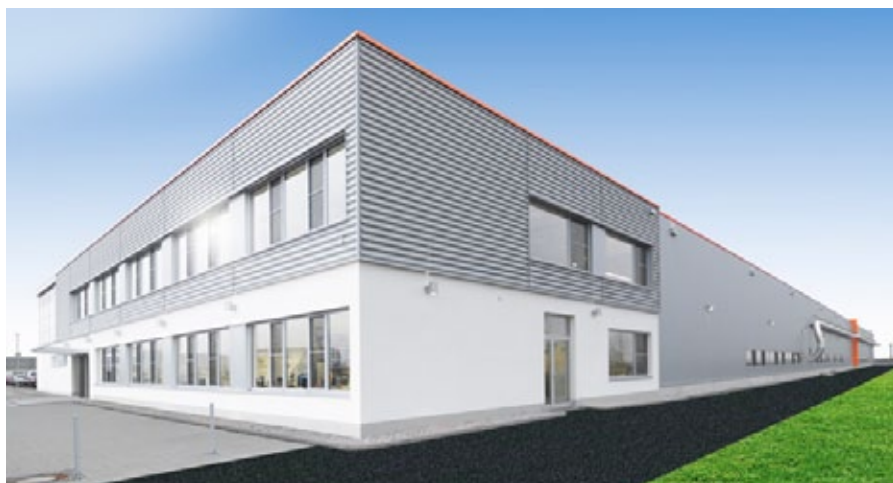
The new Panther Display works in Wustermark.
